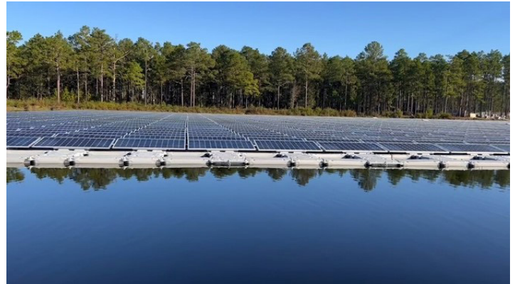
1.1 MW floating solar array with battery storage at Camp Mackall provides approximately half the site's power and provides more time for utility repair crews to respond in the event of an outage, helping to improve power reliability and resilience.
