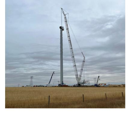
A crane at the Garden Plain wind project site stands by waiting for a window when the wind will drop low enough to start lifting. The very thing that makes building a utility-scale wind farm on the wide-open prairie so challenging is the same reason TransAlta is here in the first place: strong and steady winds.
