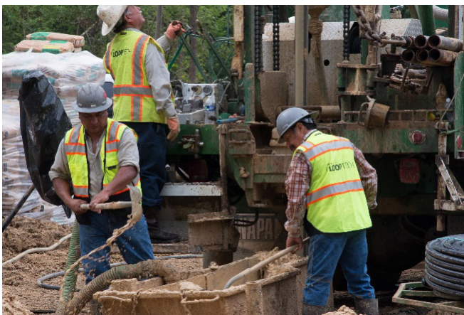
Figure 7. HARC's GSHPs use Houston's near-constant, below-ground temperature of about 72°F (Olgun 2015) to dispel or absorb heat. Photo: HARC
